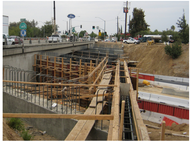
Measure T Tier 1 Project: State Route 145 widening at State Route 99 interchange.
