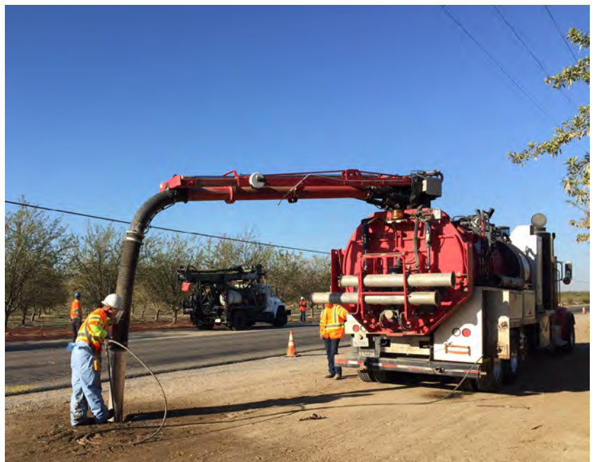
Pre-construction activities getting underway Construction Package 4 in October with “pot holing”. During this process crews locate utilities to in order to avoid them during construction. In some cases, utility relocation is necessary.
