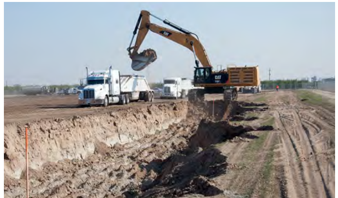
The first construction work in Construction Package 2-3 getting underway in November 2016 with the building of a test berm in Fresno County. Crews in CP 2-3 have also been busy with several road paving projects.
