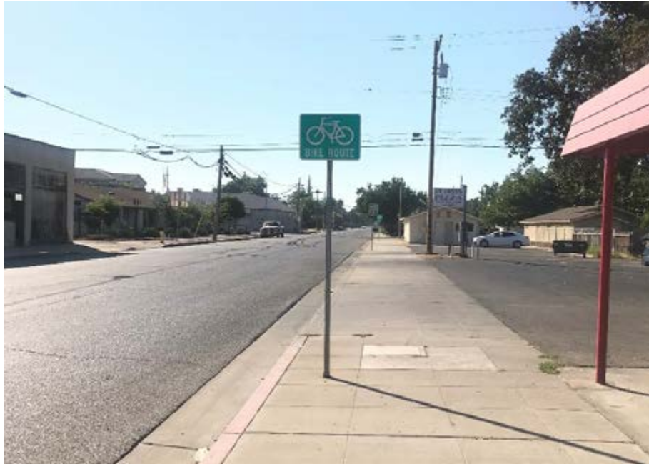
Class III Bike Route is efficient on S. 5th Street, a minor roadway with light traffic and low speeds.
