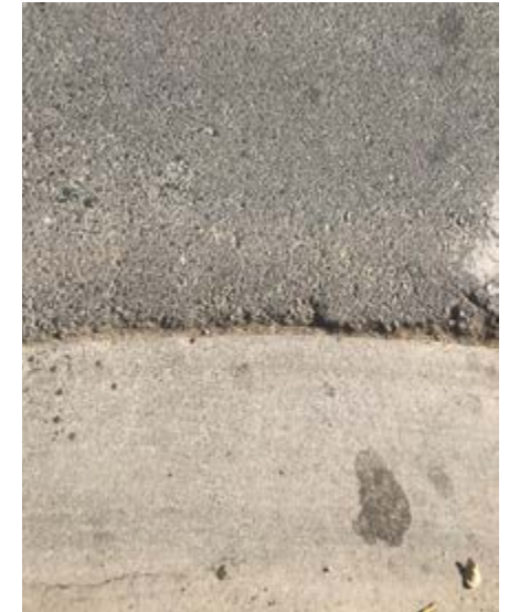
Aggregate Polishing on Robertson Boulevard near 5th Street
