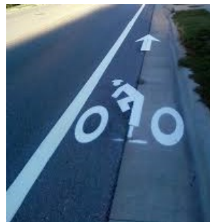
Bicycle lane painted over gutter pan
