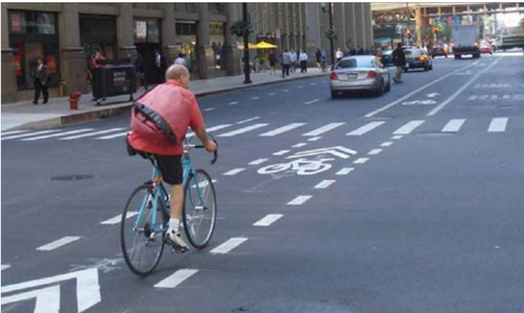
Intersection Crossing Markings
