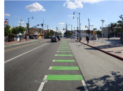
Green skip-striping at intersection where cars may merge across or into the bicycle lane
