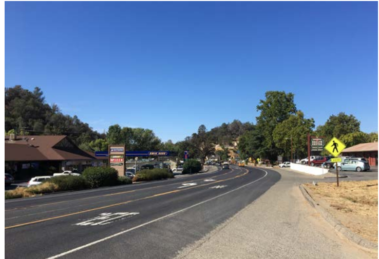
Example Enhanced Bicycle Route in Coarsegold with wide multi-use shoulders. Upgrades could include intermittent rumble strips.
