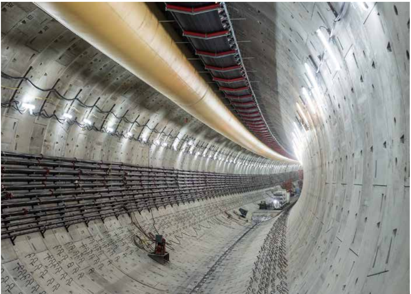
Photo credit: Washington State Department of Transportation
