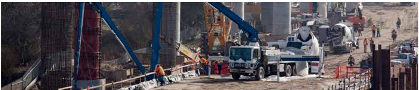
San Joaquin River Viaduct Construction in Fresno
