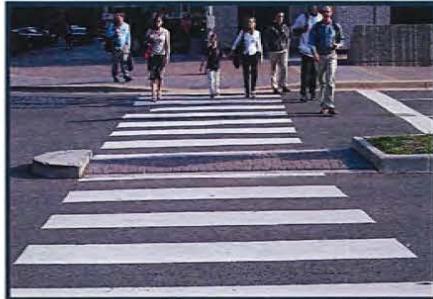
Marked pedestrian crossing Pasarela peatonal marcada
