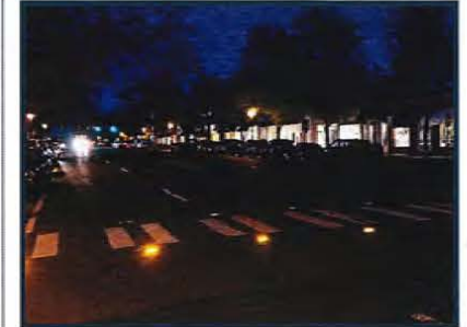
Illuminated pedestrian crossing Pasarela peatonal iluminada
