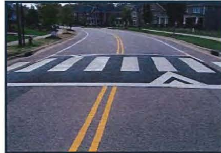
Raised pedestrian crossing Pasarela peatonal elevada
