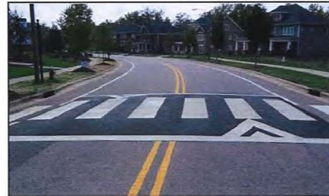
Figure 3.1 - Preferred Pedestrian Crossing Design: Elevated Crossing
