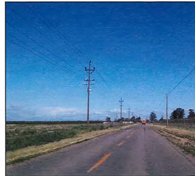
Photograph 1: Avenue 9 westward view; Source 4-Creeks 3/27/17
