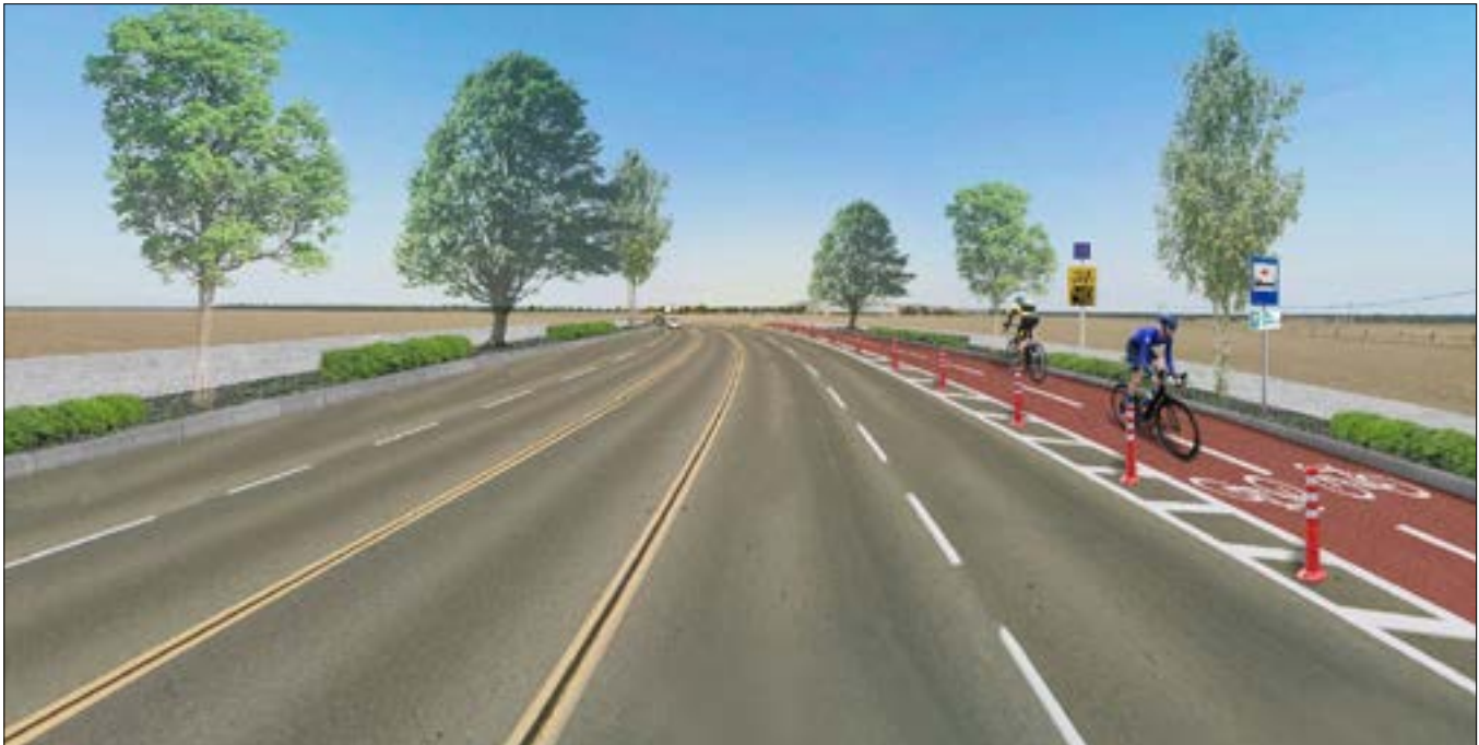
Figure 5.11: Avenue 9 Widening and Protected Bicycle Lane
