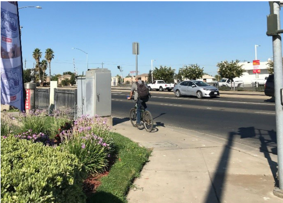
Class III facility on Robertson Boulevard at Chowchilla Boulevard. This facility does not accommodate all cyclists, due to high traffic volumes and high truck traffic in this area.AA
