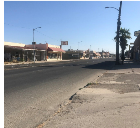
Sidewalk is not maintained near intersection of Robertson Boulevard/5th Street.
