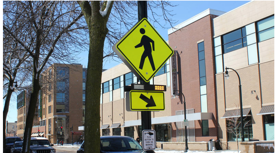
Rectangular Rapid Flashing Beacons
