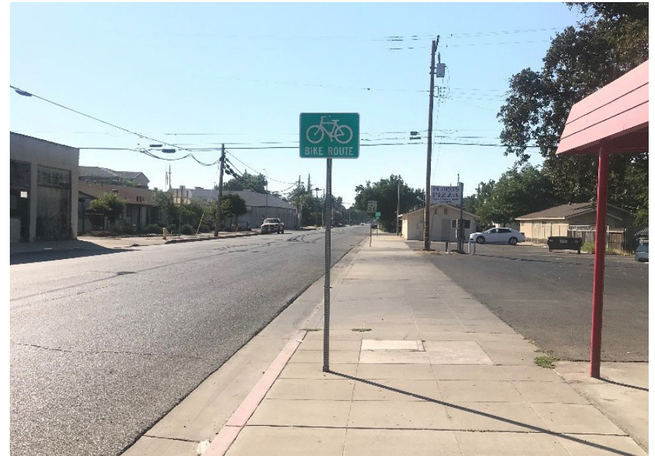
Class III Bike Route is efficient on S. 5th Street, a minor roadway with light traffic and low speeds. AA
