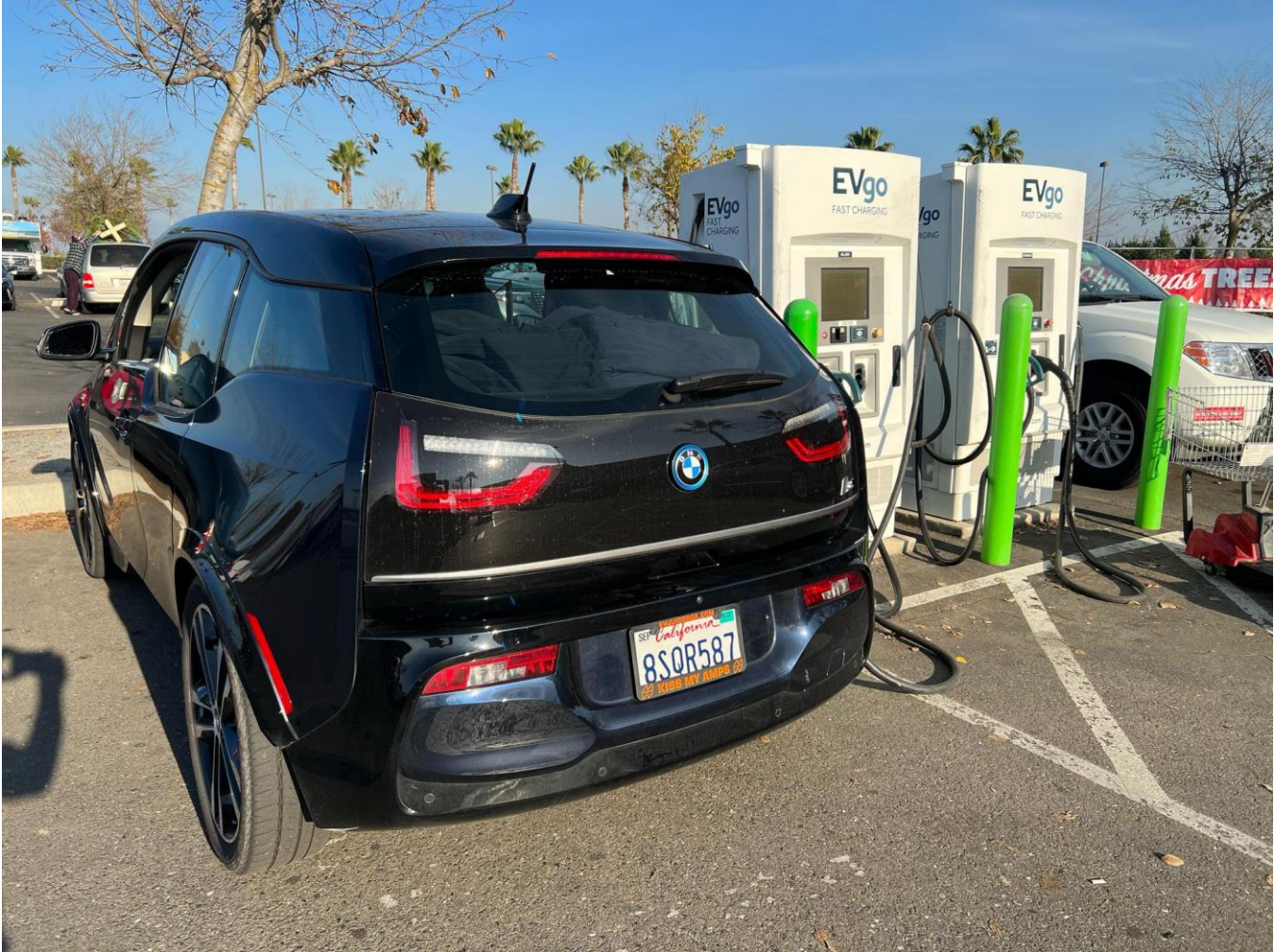
FIGURE A-8: 2 EVGO DC FAST CHARGERS, HIGHWAY 99 EXIT 170, CHOWCHILLA (PHOTO: PLUGSHARE)
