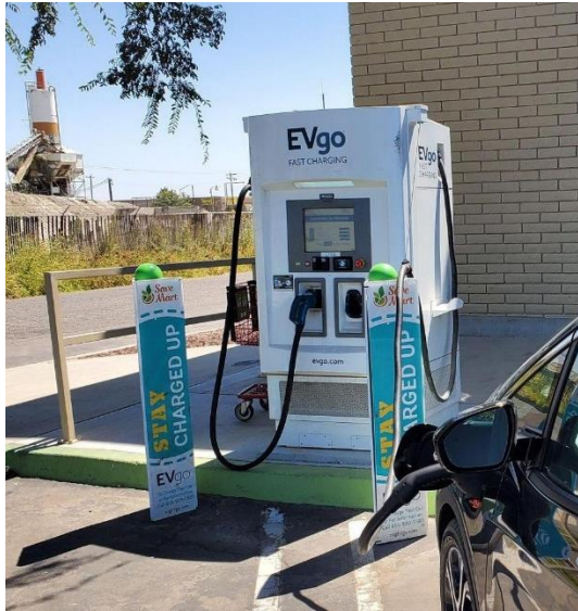
FIGURE A-2: PUBLIC DUAL-PORT DC FAST CHARGER (PHOTO: PLUGSHARE)
